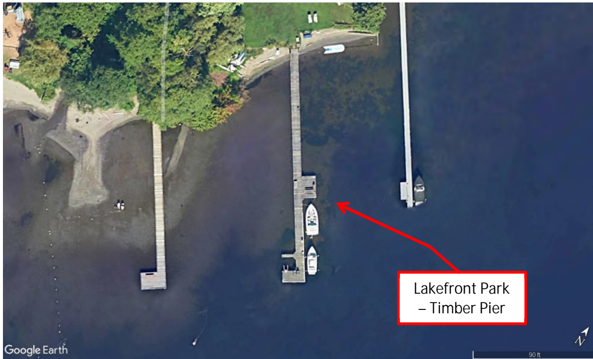
Figure 2 Aerial view of the LFP Lakefront Park timber pier
