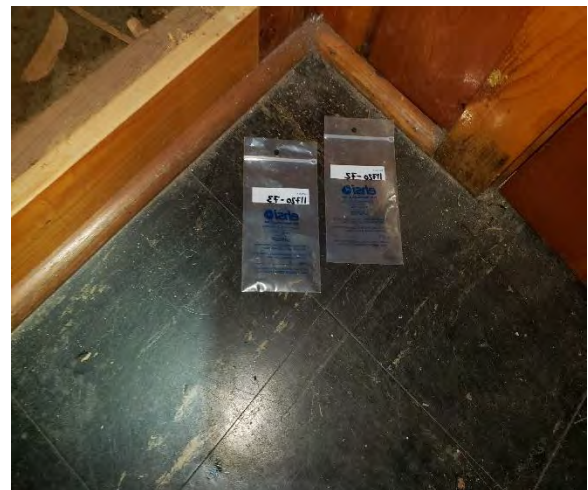
Photo #12: Samples 11720-72 & 73: 9"x9" Black VFCT on black mastic (on wood.) (4% Chrysotile) Location: Building 6 Bedroom
