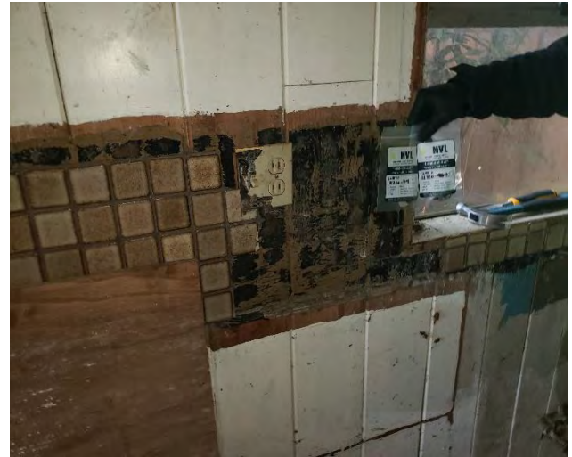
Photo #6: Samples 11720-44 & 45: 2"x2" Olive ceramic tile on yellow mastic on black mastic and 4"x3" white ceramic tile with yellow mastic (on wood.) (2% Chrysotile) Location: Building 9 Shower Area
