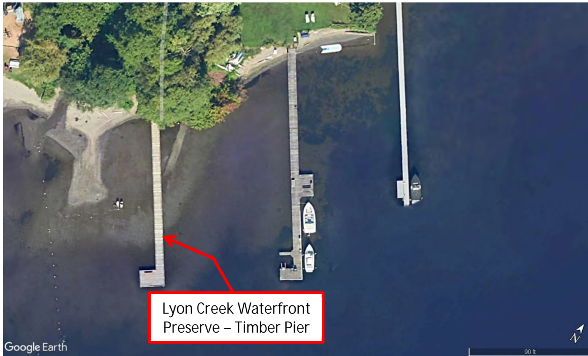
Figure 3 Aerial view of the Lyon Creek Park timber pier
